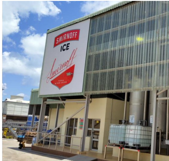
UBL RTD Plant
